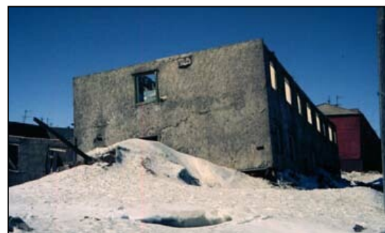
Examples of infrastructure damage caused by permafrost melting.
